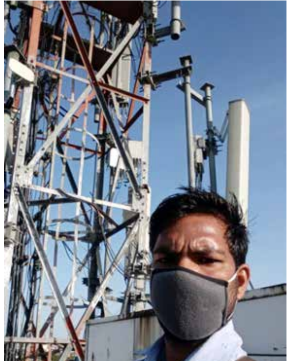
Maintenance activities continued during lock down period
